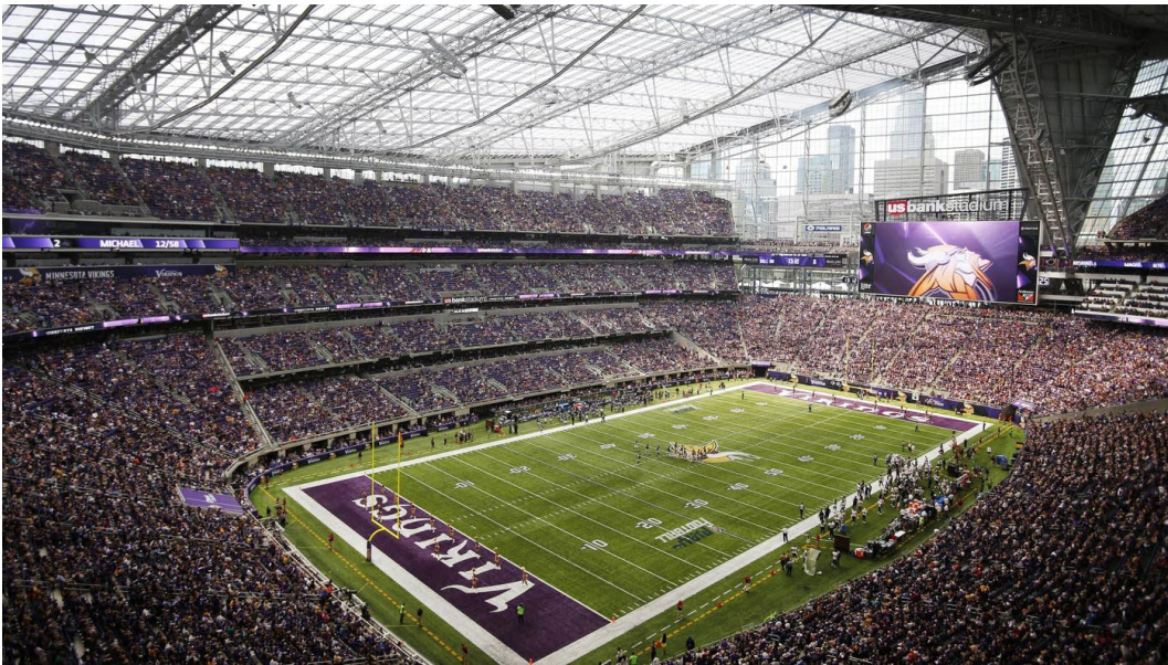
U.S. Bank Stadium, Minn., MN, 2016, HKS, Inc.. Photo: Andy Clayton-King, AP. 5
