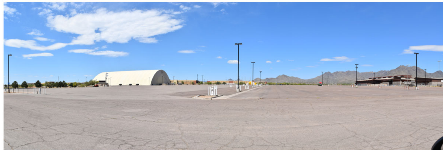
View from the Southeast
